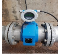
Figure 3.1: Output meter according to electromagnetic principle Endress Hauser
