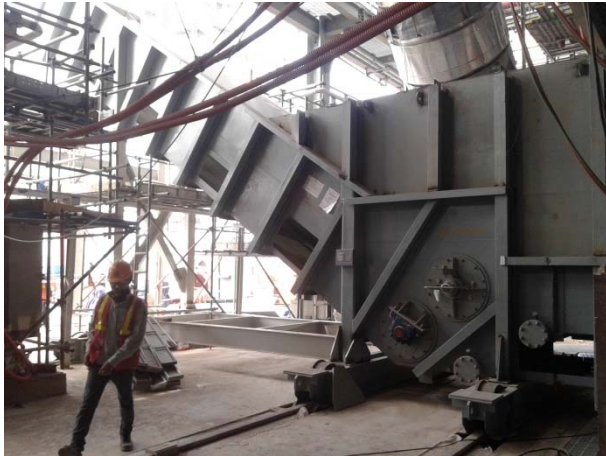
Bent Section & Ramp Section
